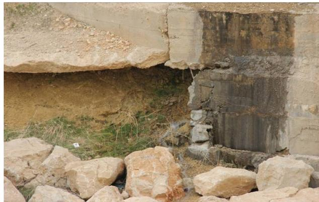
**Figure 2 : piping hole and seeping flow between abutment and concrete body**
