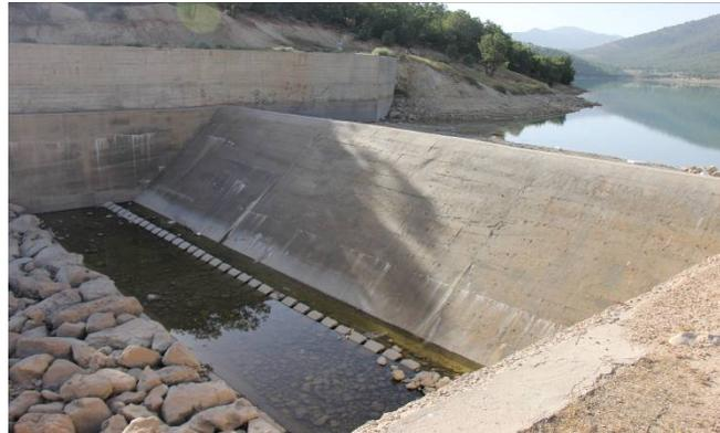
**Figure 1 : Ogee spillway of Shahghasem dam**
